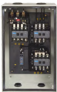
Interior View of MU FASD
