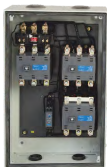
Interior View of ML FASD
