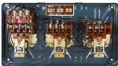
Interior View of MK2 SASD
