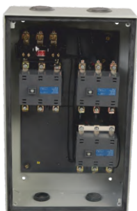
Interior View of ML SASD
